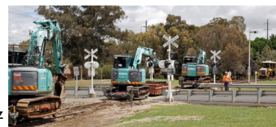
Work on the sleeper replacement at the Kandos level crossing
