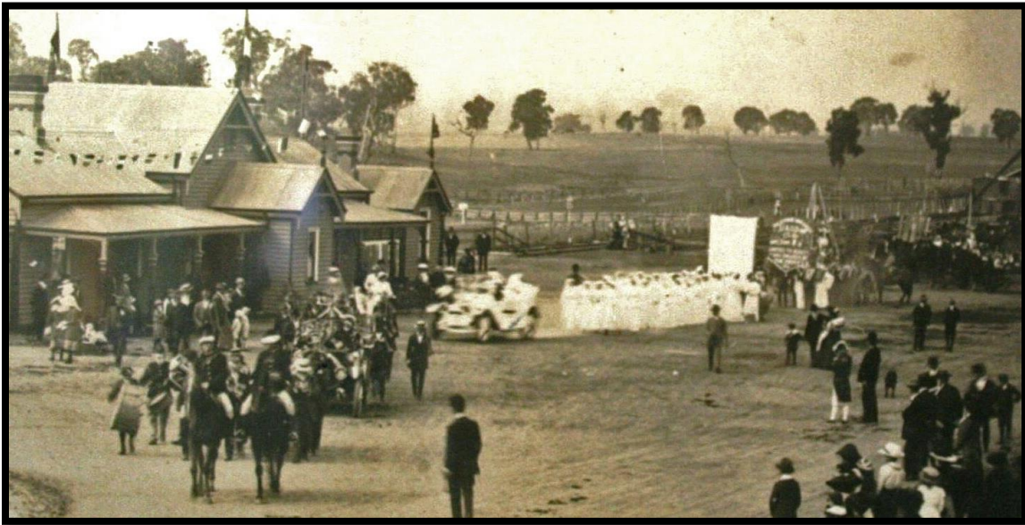
The Rylstone Australia Day Procession leaving Rylstone Railway Station 30 July 1915
